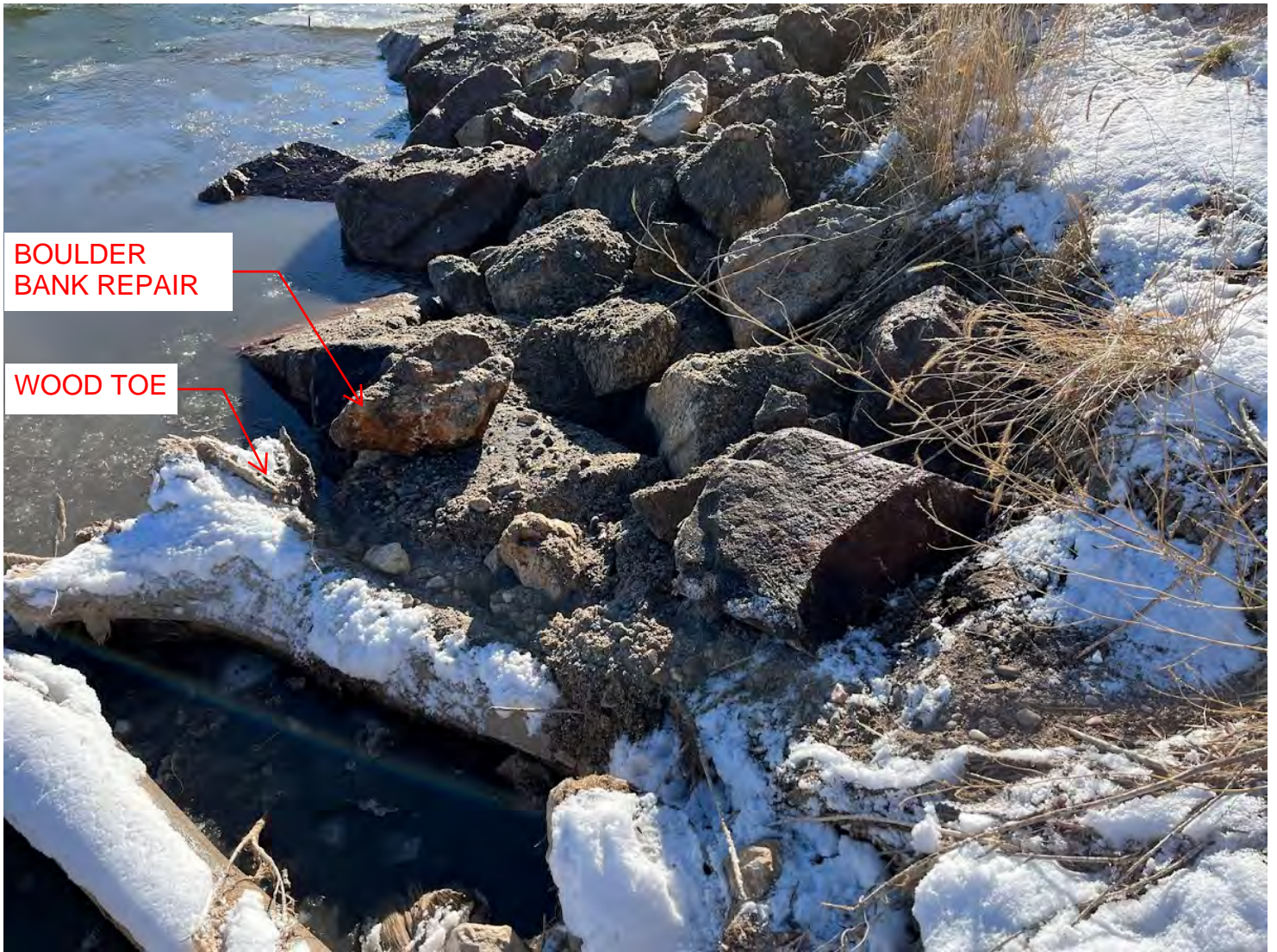
Figure 5: Boulder tie-in to wood toe structure.
